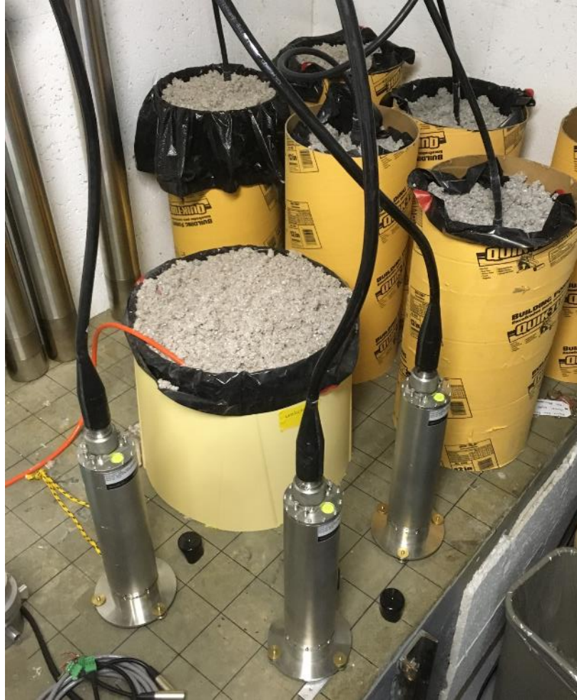
Figure 5 Picture of installed Seismometers
