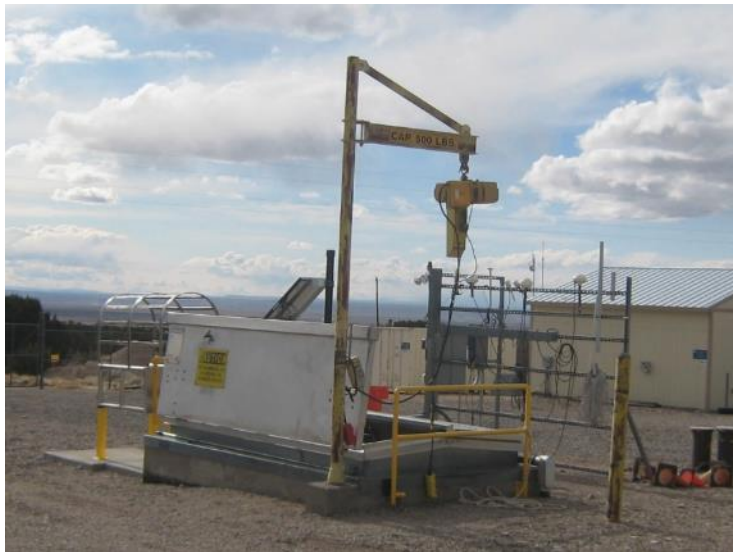
Figure 2 FACT Site Bunker
