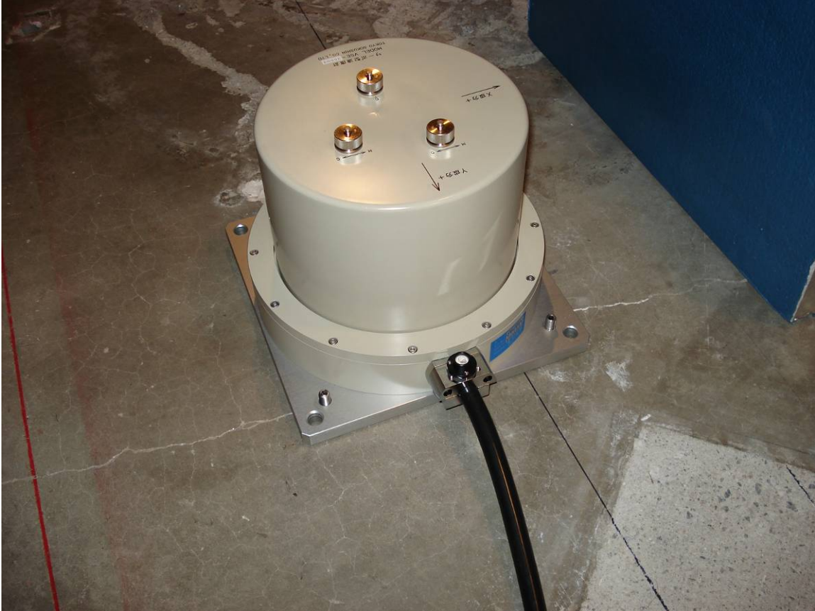
Figure 4. VSE-355G3 installed in ASL tunnel.
